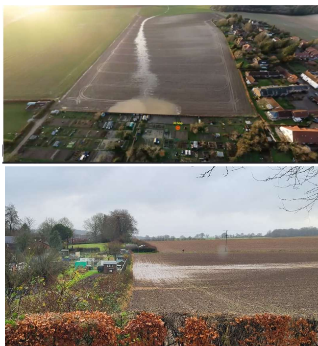
Runoff barrier in Great Bedwyn stopping flooding of home and allotments. Photo J Hitchman
